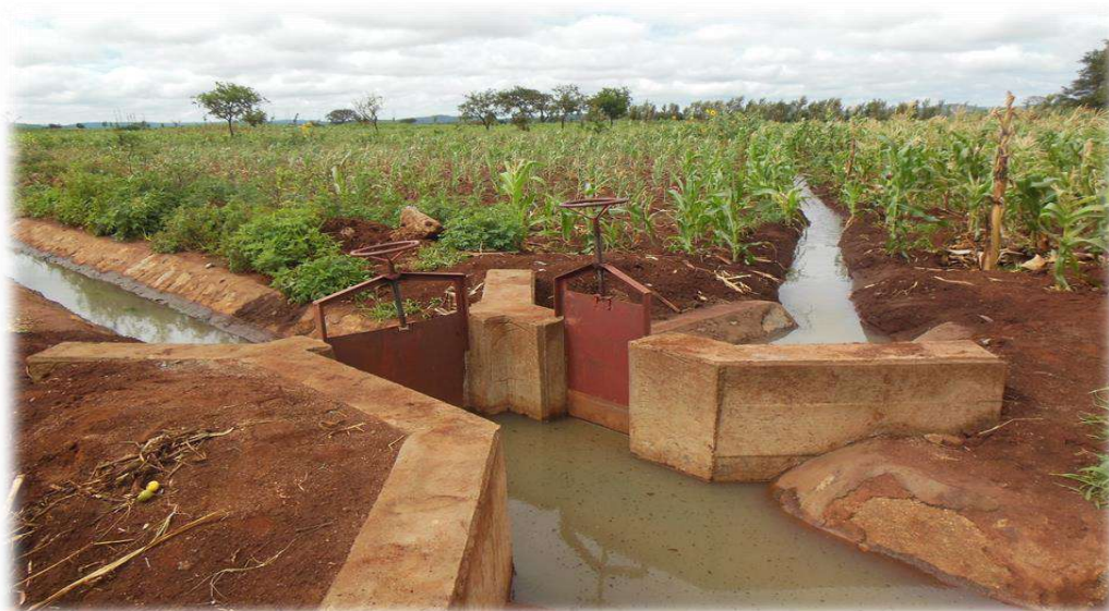
One of the division box constructed by MVIWATA
